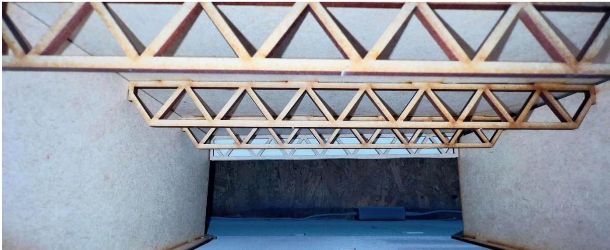
At this stage we have assembled the bridge deck with trusses and the two support structures. All that is left to do is to position the deck on the support structures. You will notice that the walls have slots where the girders will hook in. See photo above. We will leave it to you to decide whether you want to glue the deck to the supports or not.
