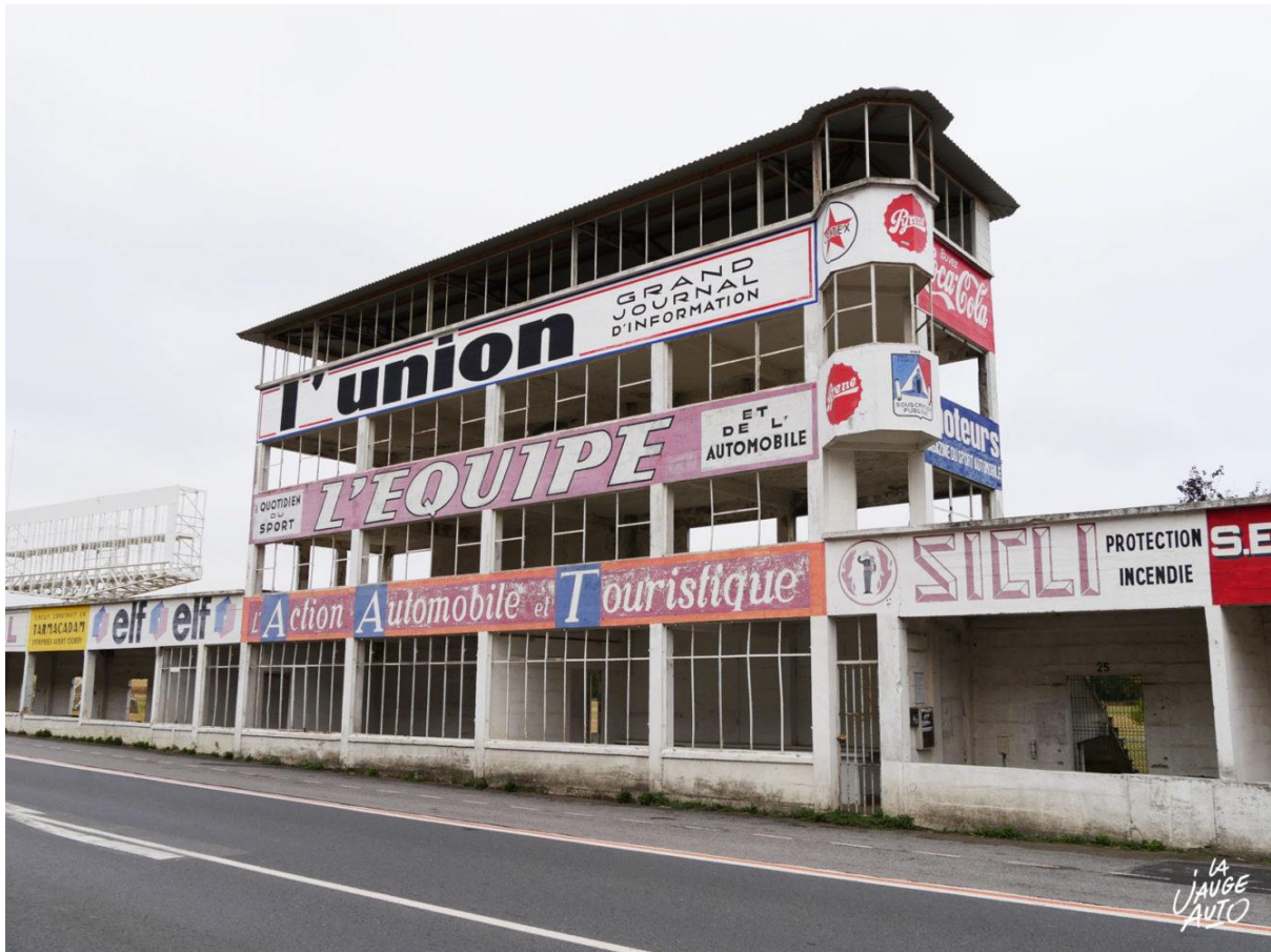
A photo of the restored building above.
